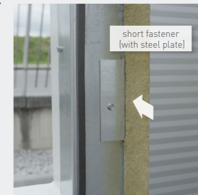
Fig. 3.6: Carrying the vertical load.
